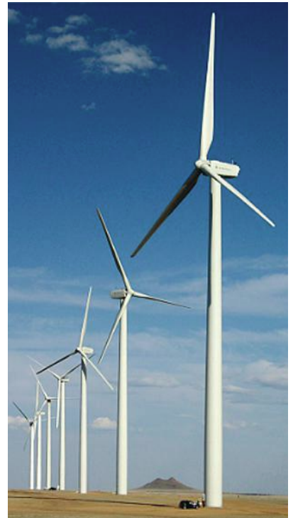
5. Wind turbines in Lamar, Colo. make up a 162-MW Colorado green wind farm. Each turbine produces 1.5 MW of electricity.
